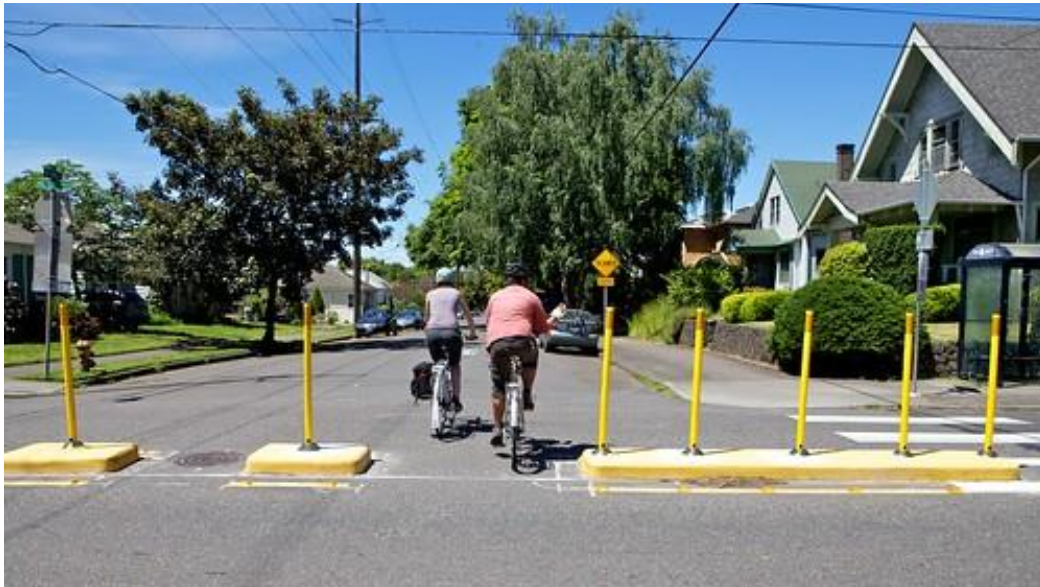
Figure 10: Median barriers restricting motor vehicle access.
