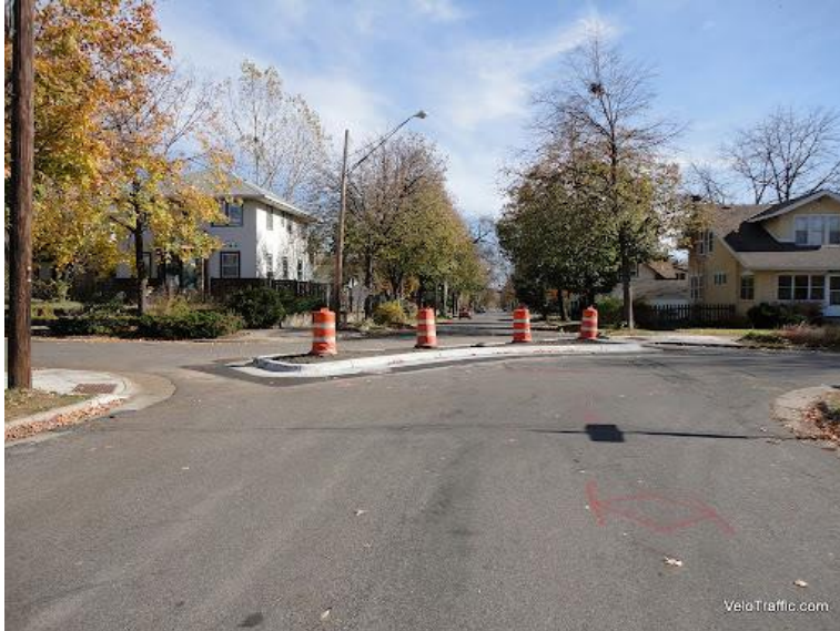
Figure 8: Diagonal diverter blocking through traffic to a residential street. Source: ITE and PennDOT
