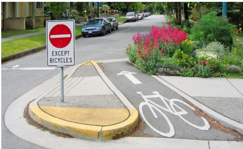
Figure 9: Half-closure blocking motorist access to a roadway. Source: Reliance Foundry
